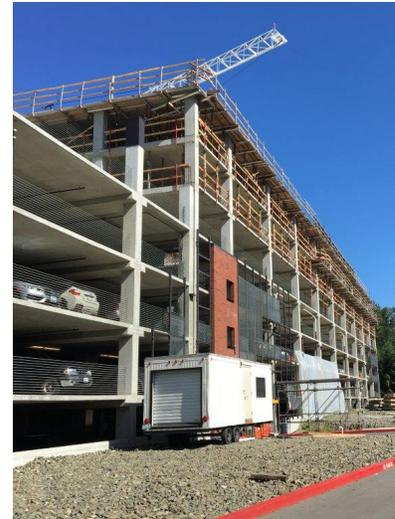
*The parking deck is being built using post-tensioned cast-in-place concrete by Ferguson Construction in Bellevue, WA.*
