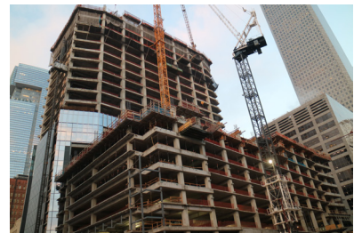
609 Main at Texas uses lightweight concrete with compressive strengths near 7200 psi.
