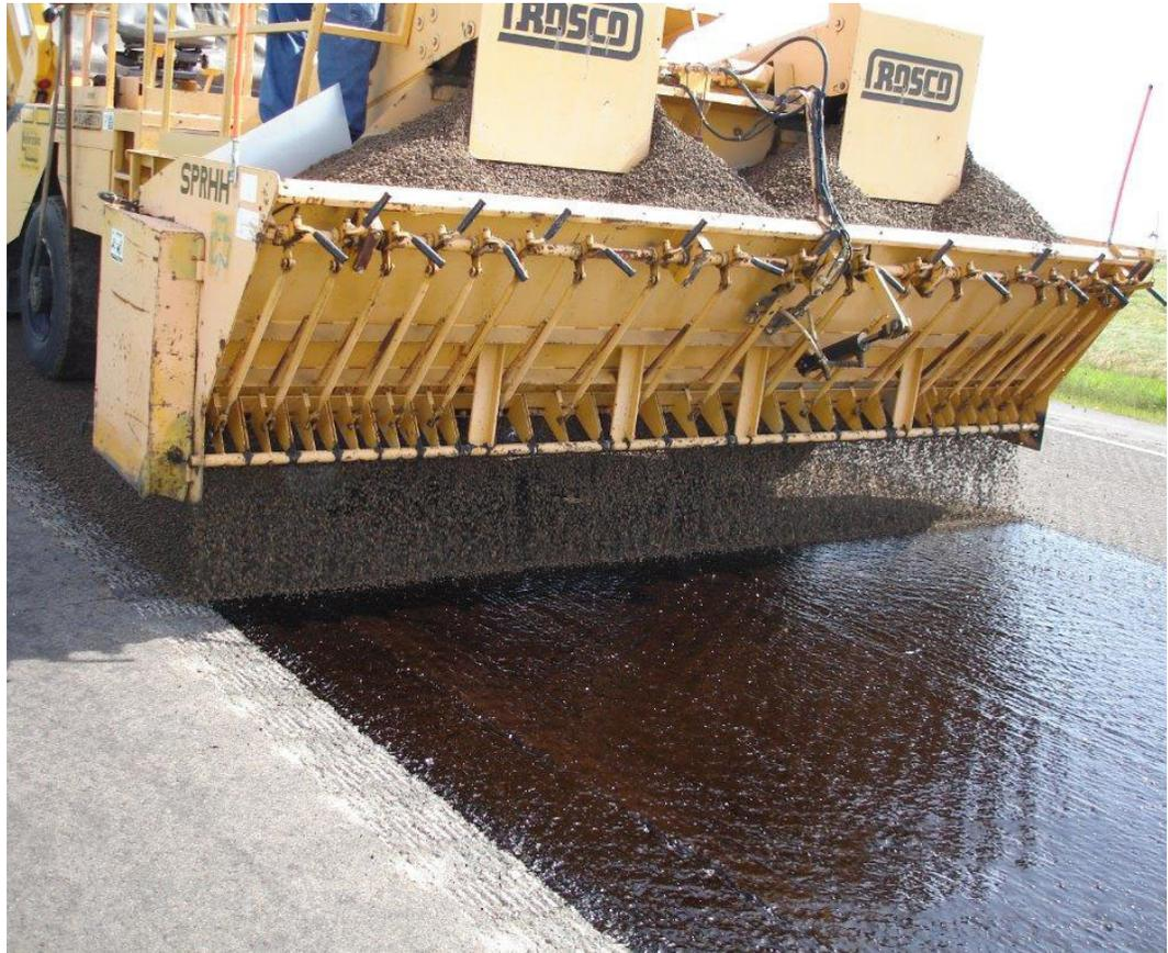
**When the Nebraska Department of Roads needed a way to economically extend the life of 6 ½ miles of pavement on State Highway 61, just south of Ogallala, they turned to a chipseal solution utilizing expanded shale lightweight aggregate from Trinity Lightweight, for both its excellent performance and its economical cost.**
