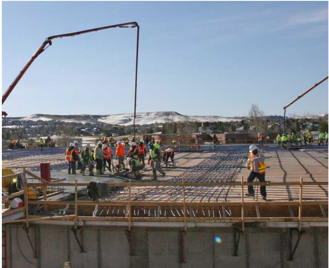
**Constructing large capacity water storage tank slabs without construction joints is a complex proposition in Colorado’s low humidity and often windy climate. One solution that has been successful is to specify low-shrinkage concrete mixtures and monolithic placement of the slab within a prescribed time period to reduce the probability of shrinkage cracking.**
