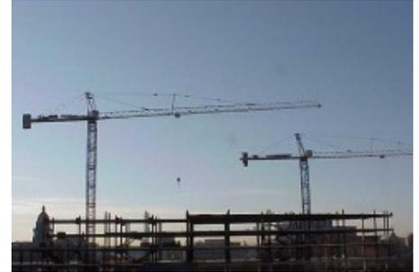
Completed in 2002, the building was constructed using lightweight concrete over metal deck. This format provided the most economical building solution to match new floor heights with the existing structure. By making it easier to pump, the vacuum-saturation of expanded lightweight aggregate product from Boulder enhanced the placement of the concrete for this project. It also offered significant dead load reduction, reduced foundation size, and created more usable space per floor.
