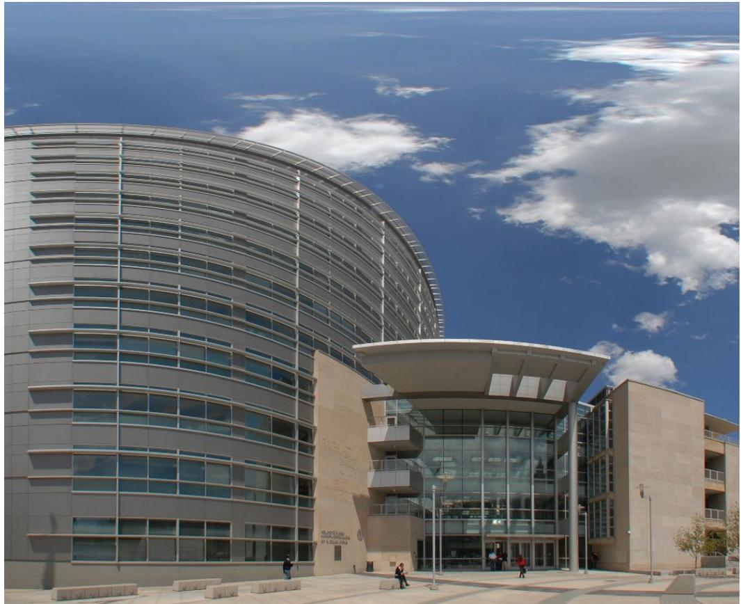
**Using more than 8,500 cubic yards of structural lightweight concrete produced with rotary kiln expanded shale, engineers constructed a 12-story addition with significant dead load reduction, reduced foundation size and more usable space per floor. Over 8,500 cubic yards of structural lightweight concrete, produced with expanded shale from Boulder, Colorado, was used to help construct an 860,000 square-foot office tower for the city and county of Denver.**
