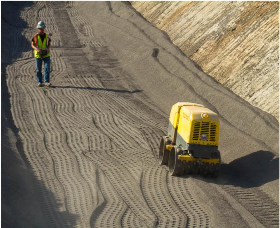
**Designers of Corridor X, a major interchange just north of Birmingham, Alabama, had an engineering challenge. New traffic lanes needed to go over the top of an existing concrete drainage system. The problem? The volume of fill material needed to build the area up to grade was enough to cause concerns about cracking the culvert.**
