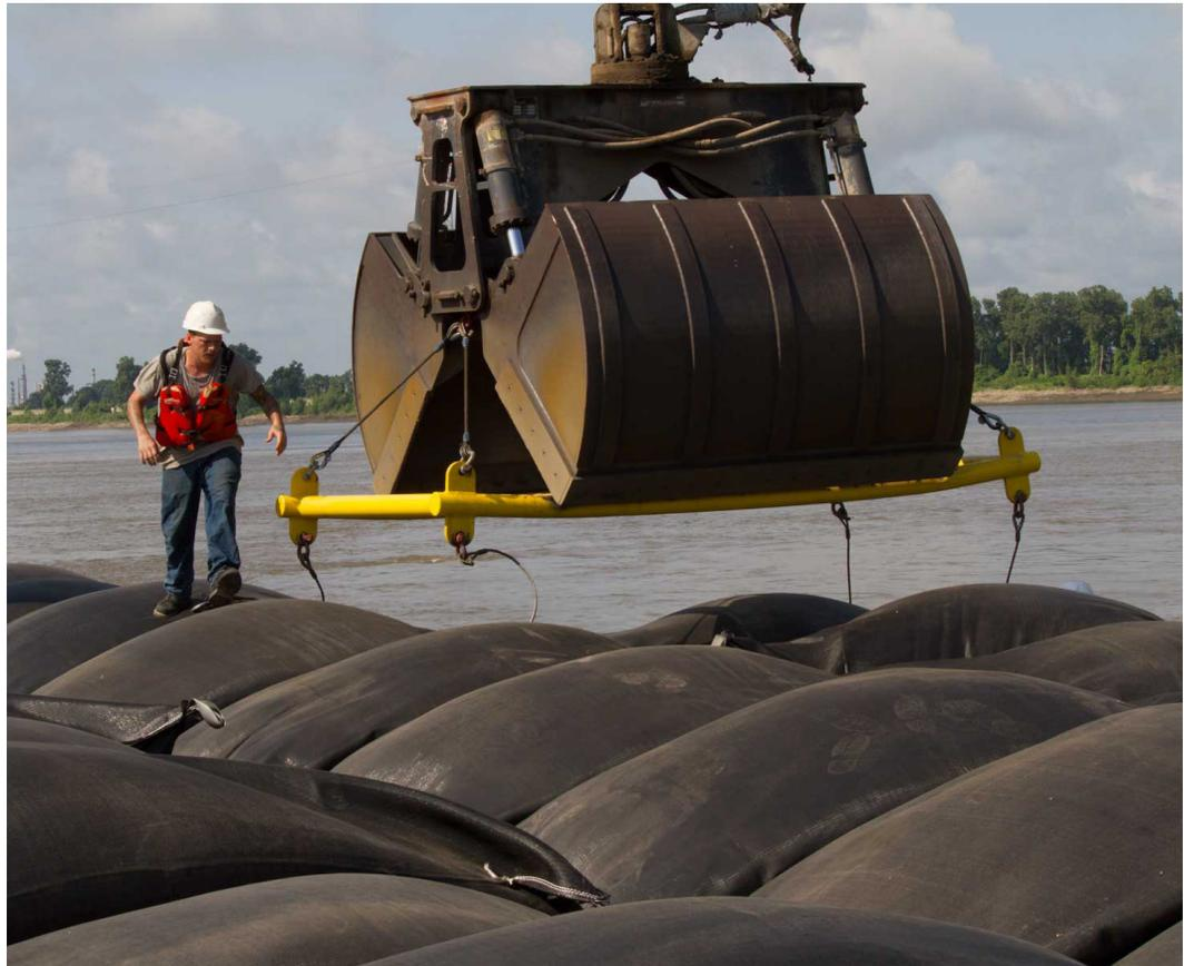
**Oversized geotextile bags filled with Riverlite® are being used to protect the shoreline and restore marshes in the Biloxi Wildlife Management Area, a vital coastal ecosystem that protects the city of New Orleans, Louisiana. The Biloxi Marsh project is located along a 7-mile stretch of the southeastern shoreline of Lake Borgne and the Biloxi Wildlife Management Area.**
